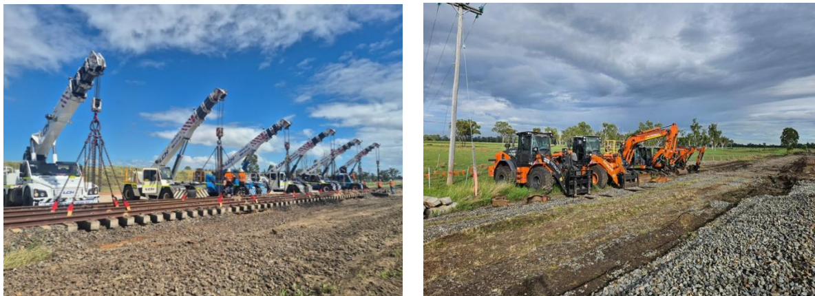
Figure 11 – 2026 Moura Flooding Repair Works
