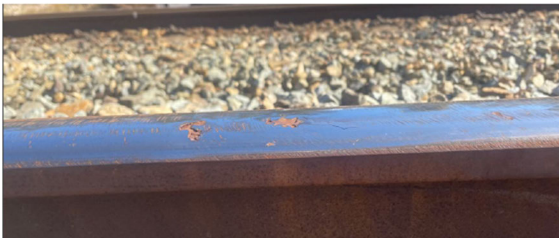
Figure 10 Turnout Hand Grinding
