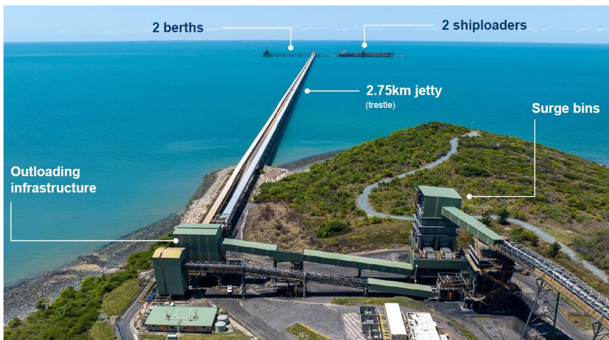
Figure 9 Terminal outloading infrastructure
