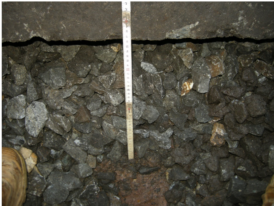
Figure 5 - Photo of ballast in sample test pit for sample 1, at 38.5km on the Down track on the North Goonyella Line, 28 July 2021. Lab PVC 3.9%
