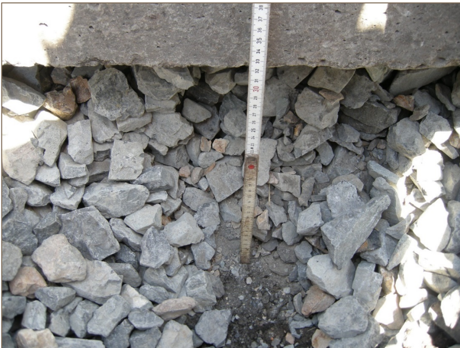
Figure 7 – Photo of ballast in sample test pit at sample site 4E, at 65.534km on the Down track on the Central Line, 26 September 2020. Lab PVC 0.7%
