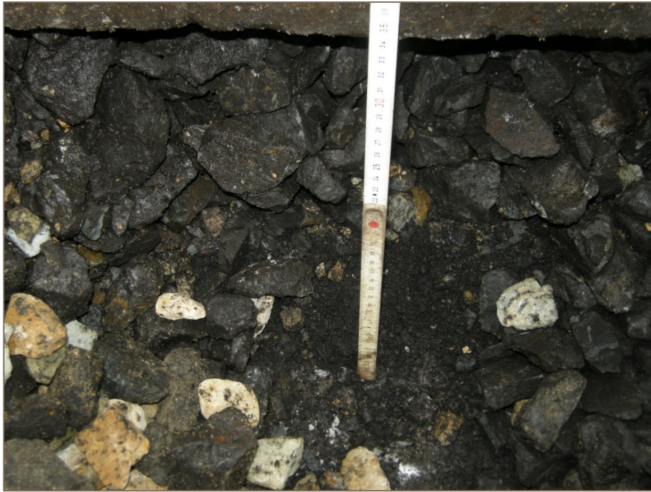
Figure 6 – Photo of ballast in sample test pit at sample site 3C, at 555.465km on the Up track on the North Coast Line, 24 September 2020. Lab PVC 18.5%
