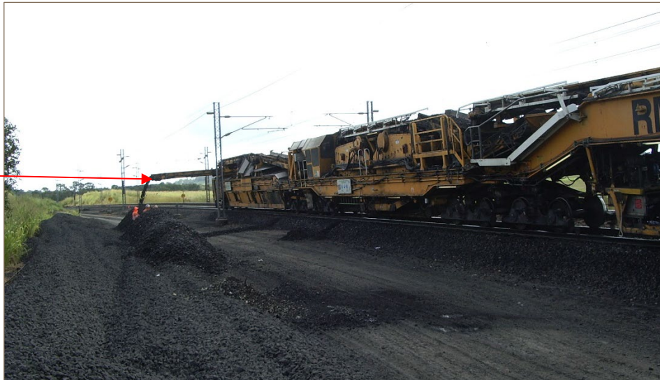
Figure 3 – RM900 discharging material (unscreenable ballast and/or screened fouling material)
