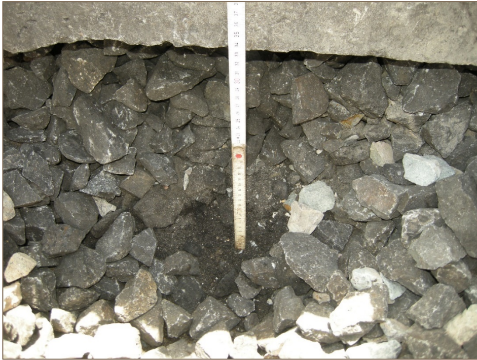
Figure 4 – Photo of ballast in sample test pit at sample site 2F, at 24.774km on the Down track on the North Goonyella Line, 14 September 2020. Lab PVC 8.6%
