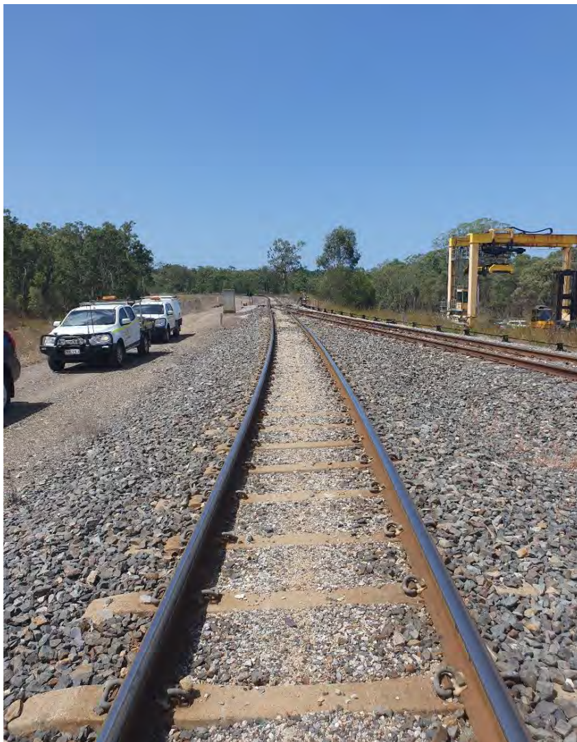
Figure 5-2 Newly replaced sleepers, fasteners, ballast, and rail
