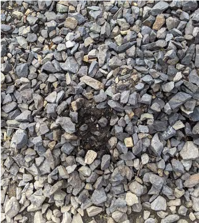
FIGURE 2 EXAMPLE TAKEN FROM SITE VISIT OF FOULED BALLAST. STONES DEGRADED AND EDGES ROUNDED (UNABLE TO “LOCK”) AND MIXED WITH COAL DUST CONSTRAINING ITS ABILITY TO DRAIN
