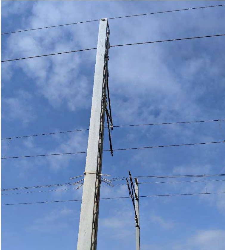
FIGURE 1 GENERALLY, THE OVERHEAD LINES HAVE A 70-YEAR LIFE SPAN. HOWEVER, SOMETIMES COMPONENTS NEED TO BE REPLACED EARLIER SUCH AS CLAMPS OR ARMS. THIS AVOIDS MAJOR RENEWALS TO THE OVERHEAD LINE. THE BUDGET IS GENERALLY BASED ON WHAT WAS DONE IN PREVIOUS YEARS.
