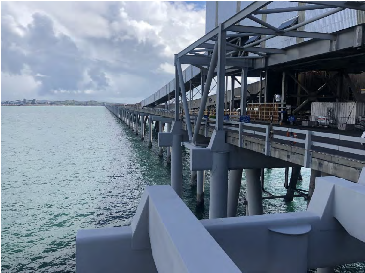
Photo 1: Offshore Domain – Jetty
