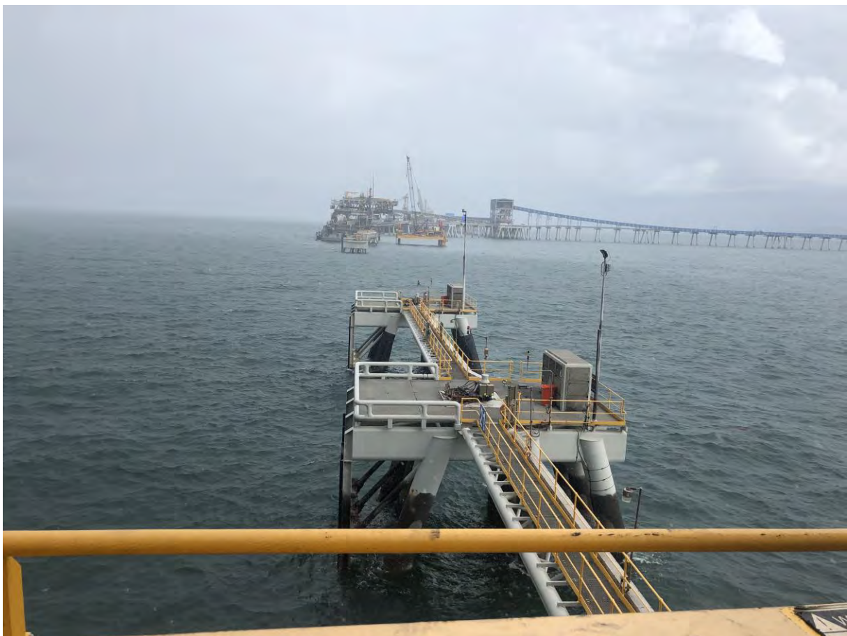
Photo 2: Offshore Domain – Jetty and wharf
