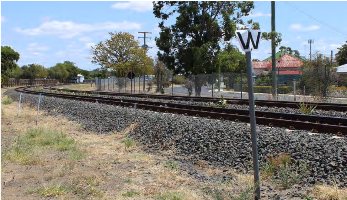
Figure 5.11. Reconstructed track at Laidley.
