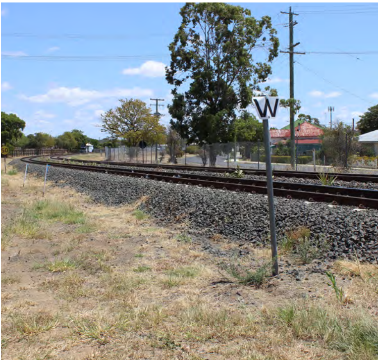
Figure 6.14. Formation rebuild R2J
