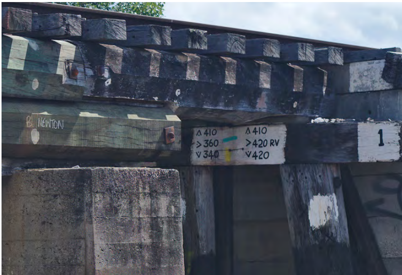
Figure 6.27. Bridge R2J Superstructure
