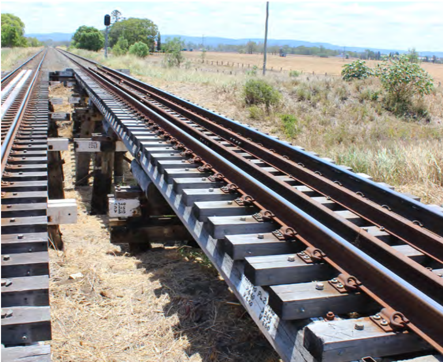
Figure 4.4. Pair of timber bridges at Kilometre 88.45, BRL_01140 and BRL_01141. Replacement of bridges will release spare components to maintain lower priority timber bridges.
