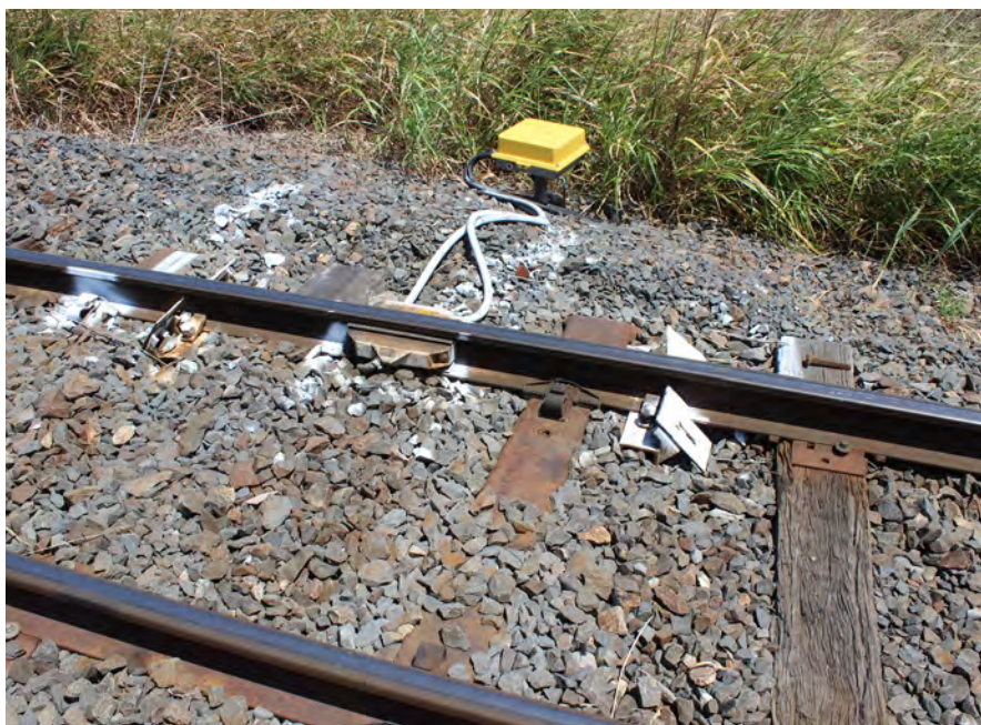
Figure 6.21. Axle counter
