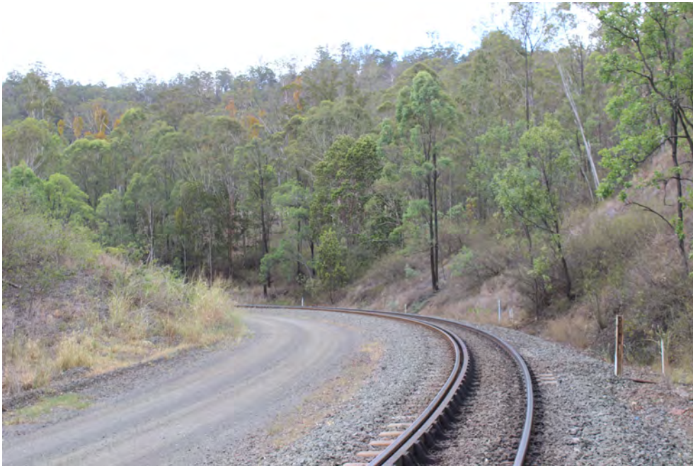
Figure 6.37. Tight curves on the Toowoomba Range; the tightest curve on the Range has an 88m radius.
