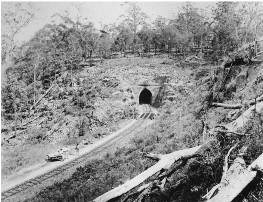
Figure 3.4. Railway tunnel on the Toowoomba Range circa 1894 17
