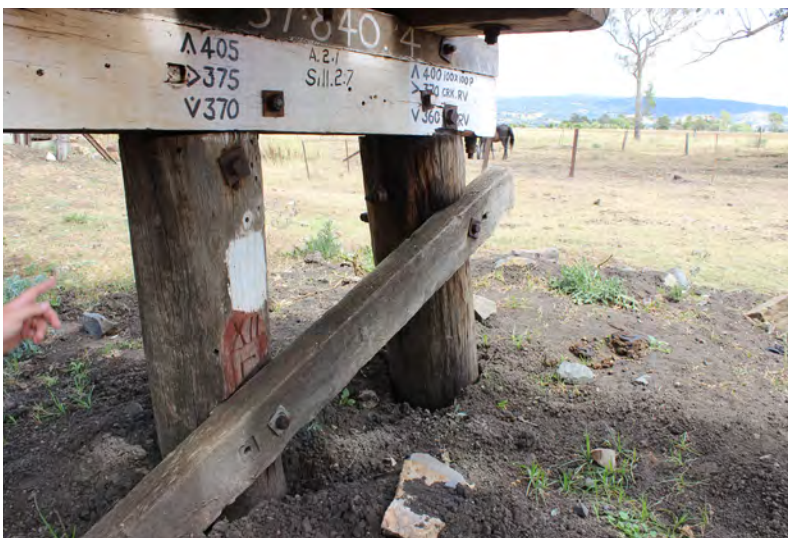
Figure 6.29. Bridge R2J - Substructure
