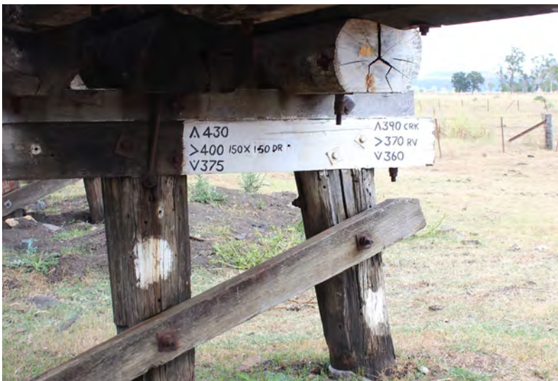
Figure 6.28. Bridge R2J Superstructure
