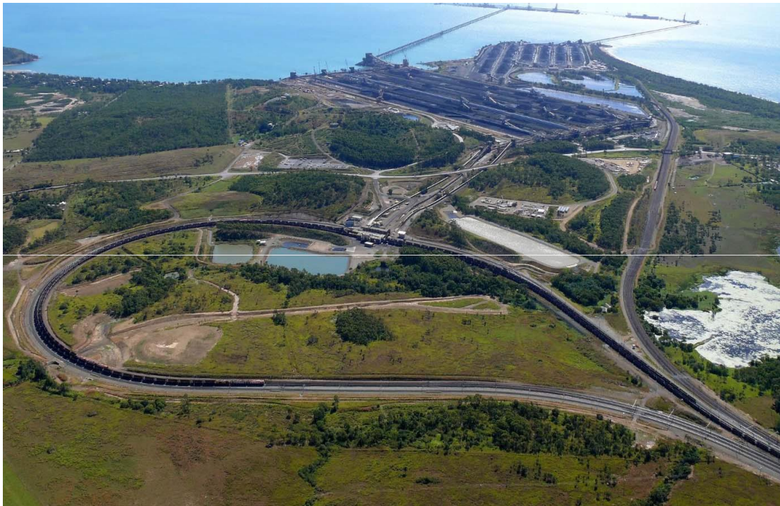
Figure 1 DBCT at the Port of Hay Point
