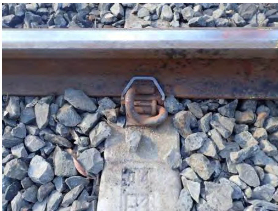
Figure 4: Worn rail in the West Moreton system
