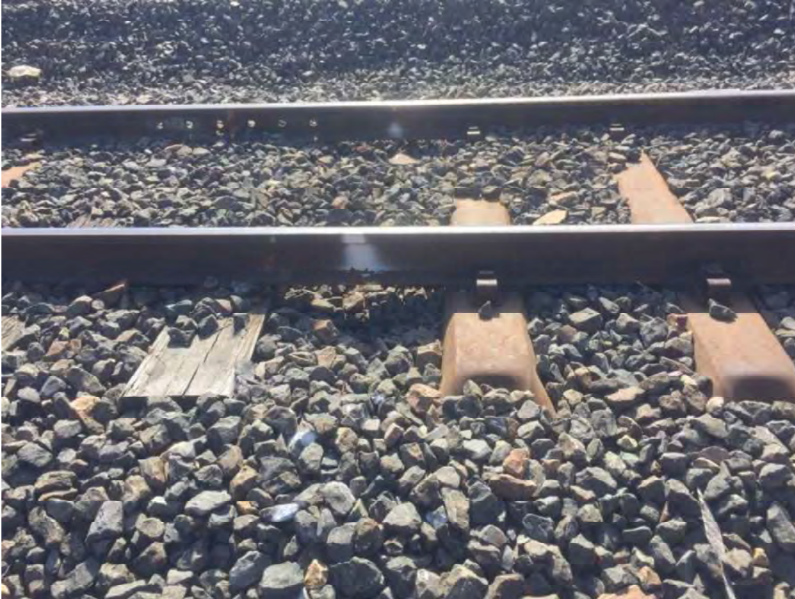
Figure 8: Mix of timber and steel sleepers
