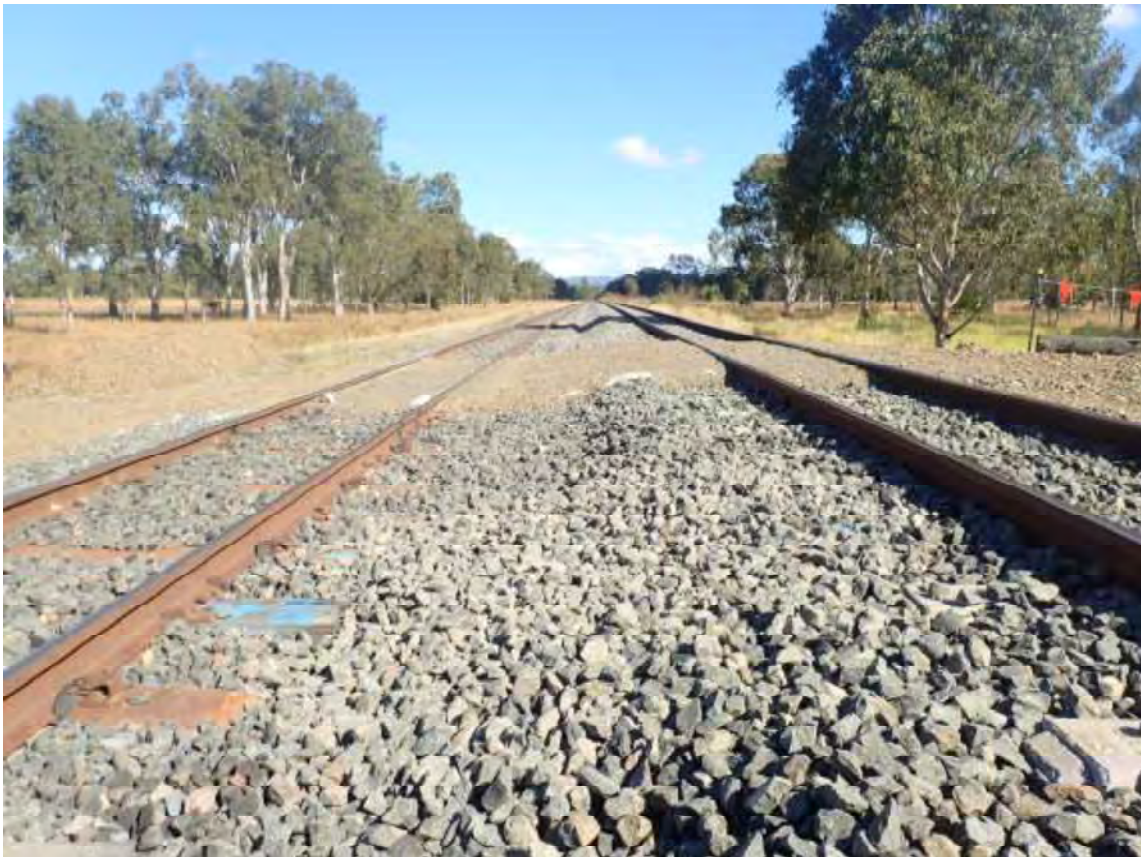
Figure 2: Recent track lowering works near Laidley on the up-road track
