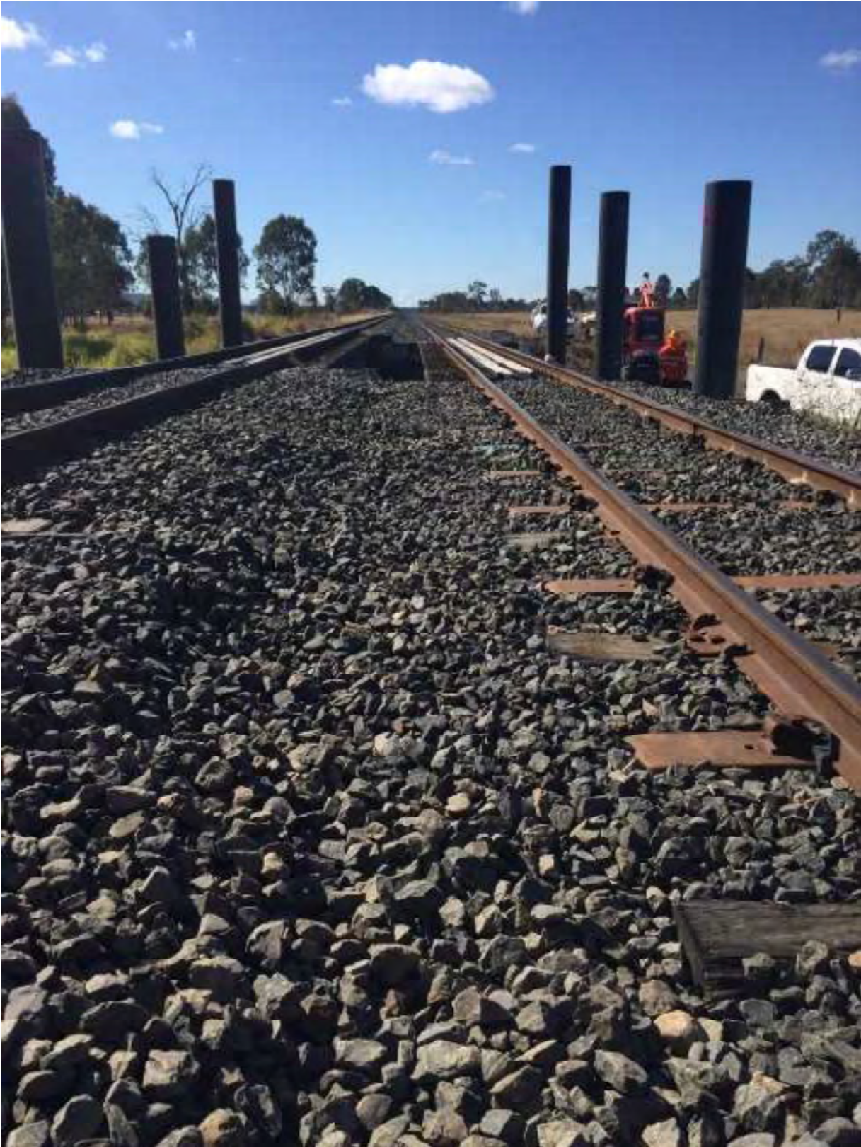
Figure 7: Use of a mix of steel and timber sleepers on parts of the West Moreton system
