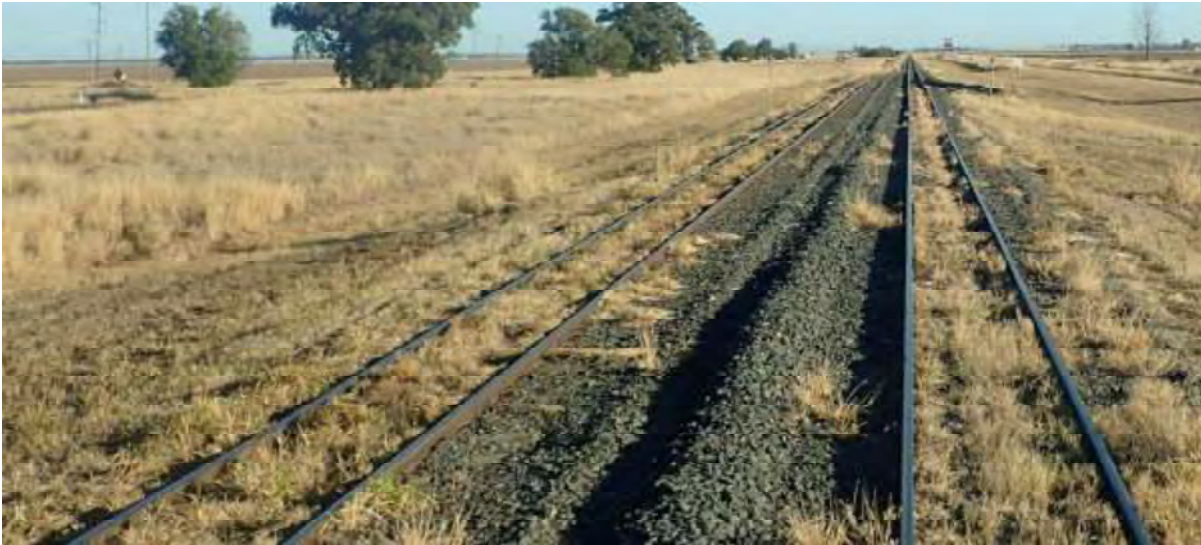
Figure 4: Dense vegetation growth through the track bed in parts of the track between Toowoomba and Miles, a symptom of the non-engineered formation characteristic of the West Moreton System
