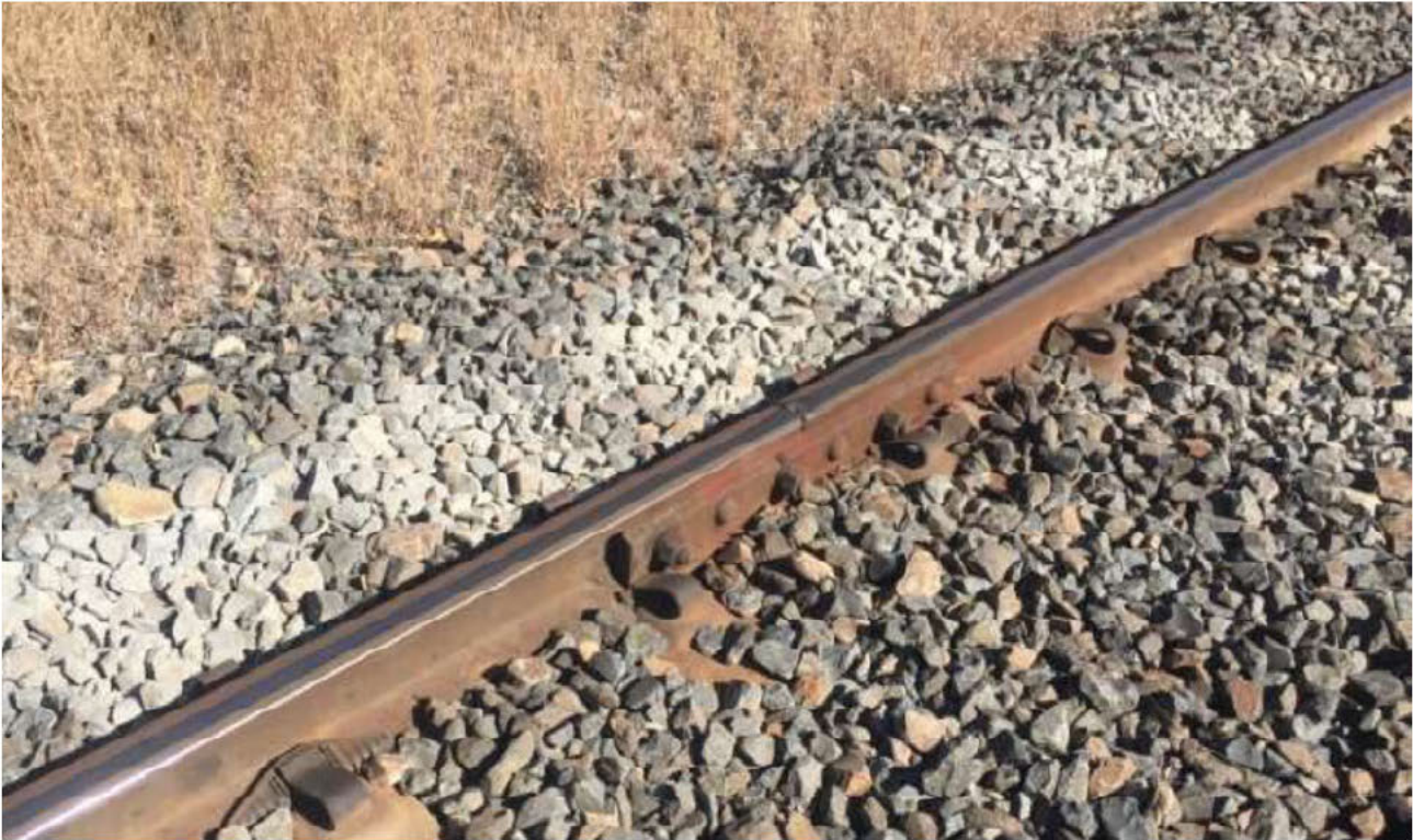
Figure 18 Battered and frozen joint
