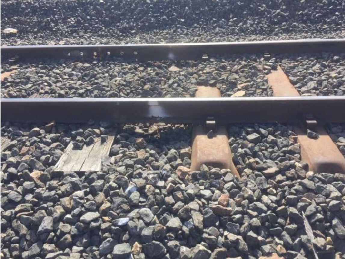
Figure 8: Mix of timber and steel sleepers
