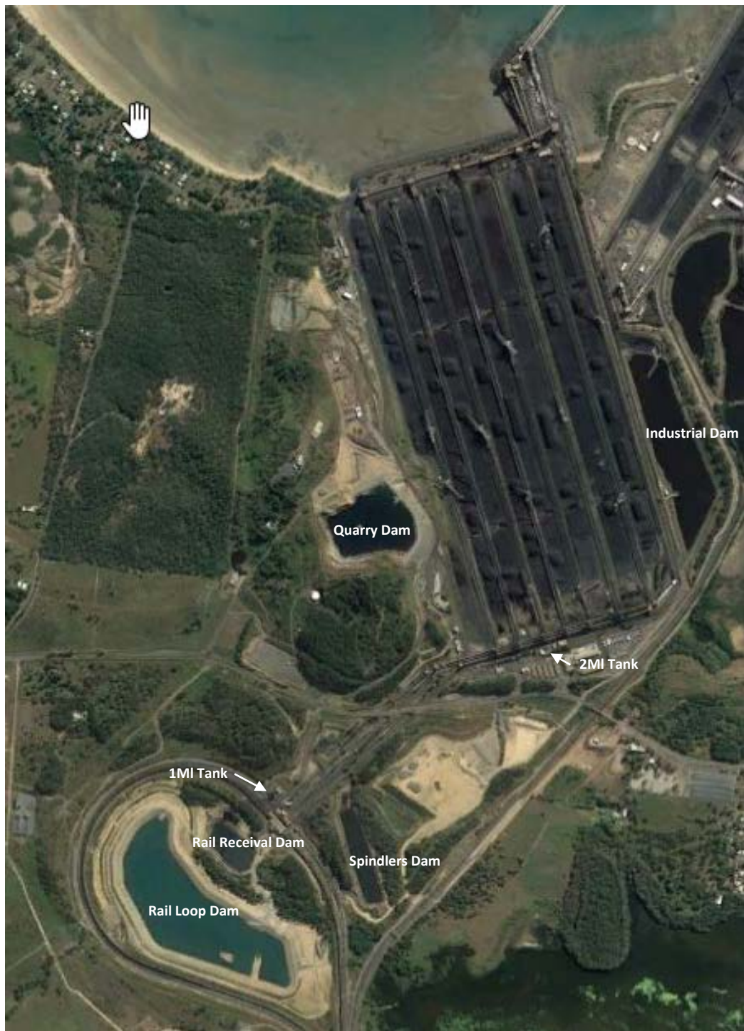
Figure 7: Water Management Infrastructure
