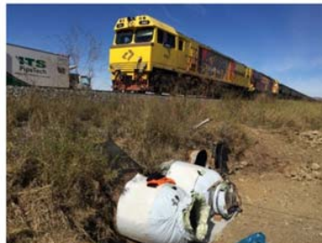
Trains running while resin installation in progress
