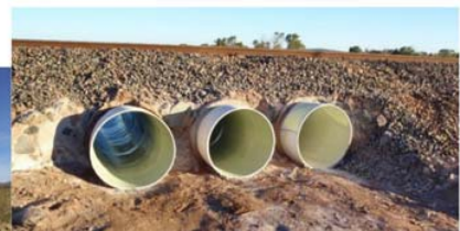
Culverts after completion of resin and fiberglass liner
