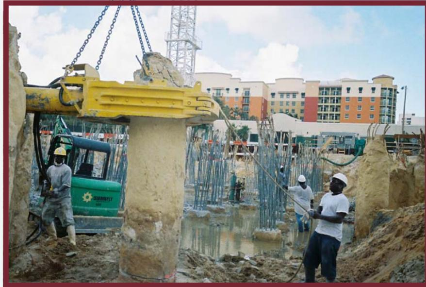
Our crushing blades fit round, square, or octagonal pre-stressed or cast in place piles from 12 inches to 36 inches in diameter.
