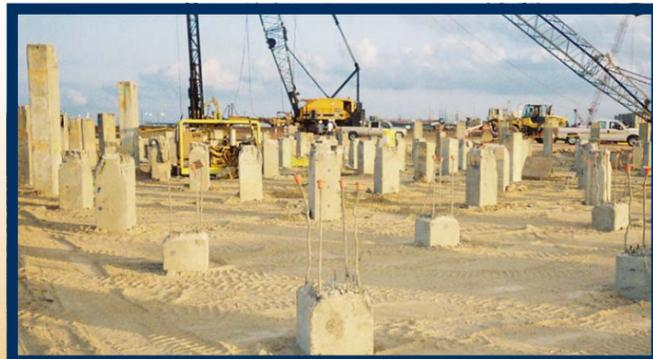
We cut piles ranging from 12 inches to 50 inches and are currently expanding our services to accommodate 60 inch piles. We commonly cut concrete precast piles, auger cast in place piles, pipe piles, and have even cut steel h-beams. We enjoy a challenge, adapting or modifying our cutter to suit specific situations.
