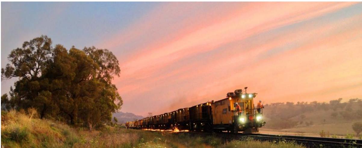
Figure 43: Rail Grinder in operation
