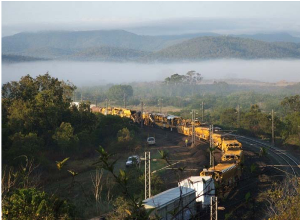
Figure 39: Aurizon Network ballast cleaning operation, RM900 ballast cleaning machine working in CQCN
