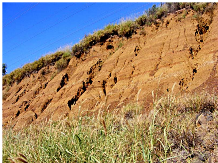
Figure 16: A cutting through sodic soil at Riverside on the Goonyella Line
