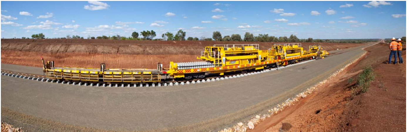
Figure 4: Track Laying Machine on the NML
