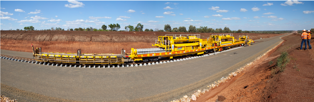
Figure 4: Track Laying Machine on the NML
