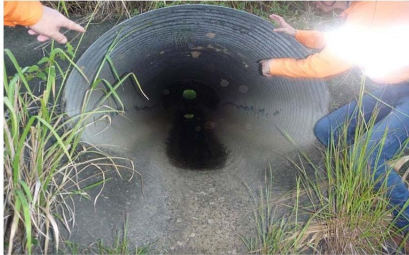
*Note: the distortion of the culvert from a circle to an oval at mid span, indicating preliminary signs of loss of structural integrity of the culvert*
