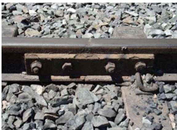
**Figure 7: Coal Dust Contamination of Track Ballast and Surrounds**
