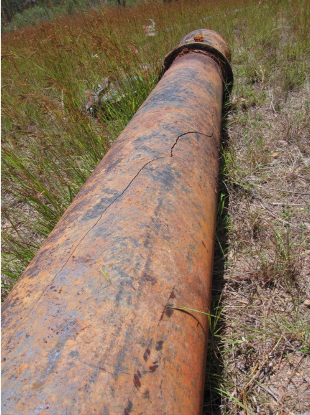
Longitudinal Failure of 300 CICL Treated Water Pipeline, Manns' Ridge
