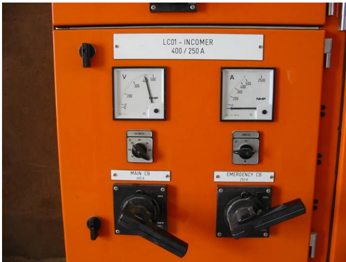
LC01 in-come/ generator change over switch
