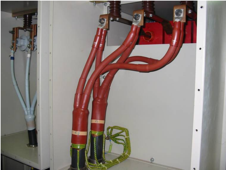
Incoming 3.3kV supply from transformer No.1
