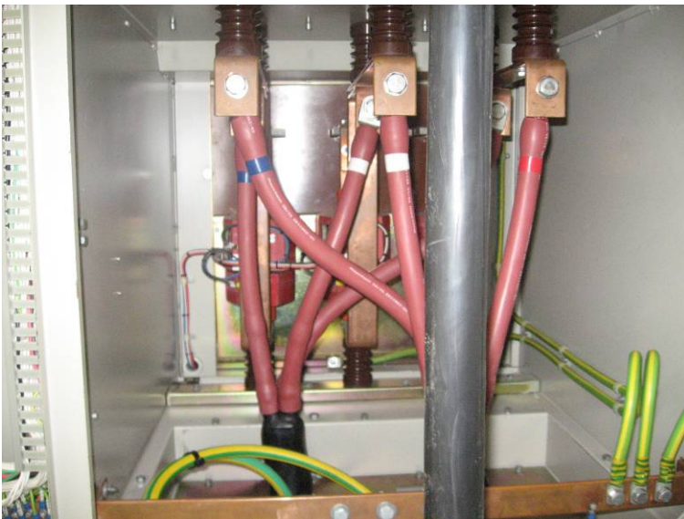
Outgoing 3.3kV supply to Pump No.3
