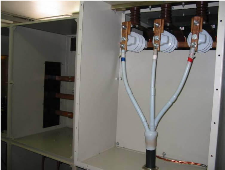
Outgoing 3.3kV supply to services transformer
