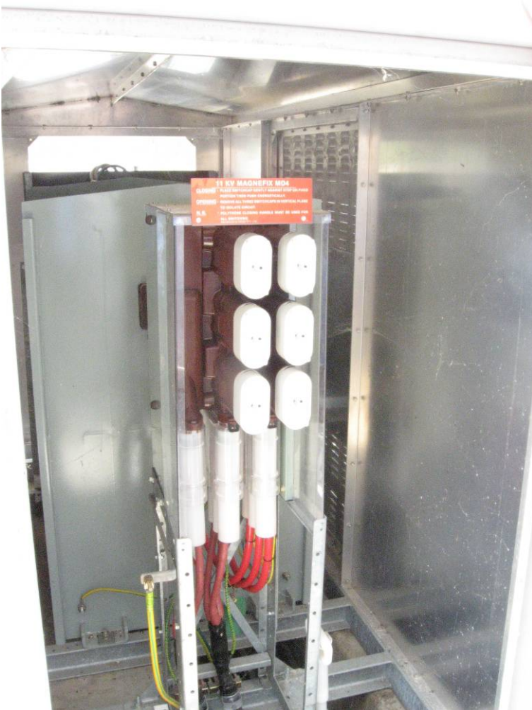
Pad mounted transformer showing 3.3kV supply from sub station entering the bottom of the isolating link arrangement. The cable leaving the centre section of the isolation links supplies 3.3kV to the Old Intake Tower. Cables leaving the right hand side links supplies 3.3kV to the primary side of the pad mount transformer.
