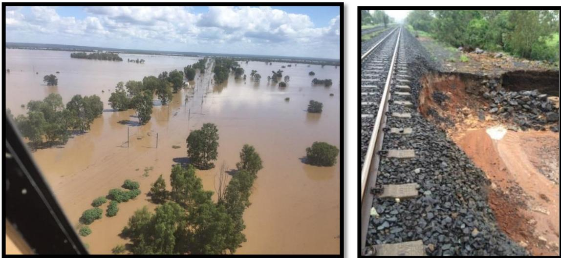
**Figure 14 – Blackwater flooding and washout / scour**
