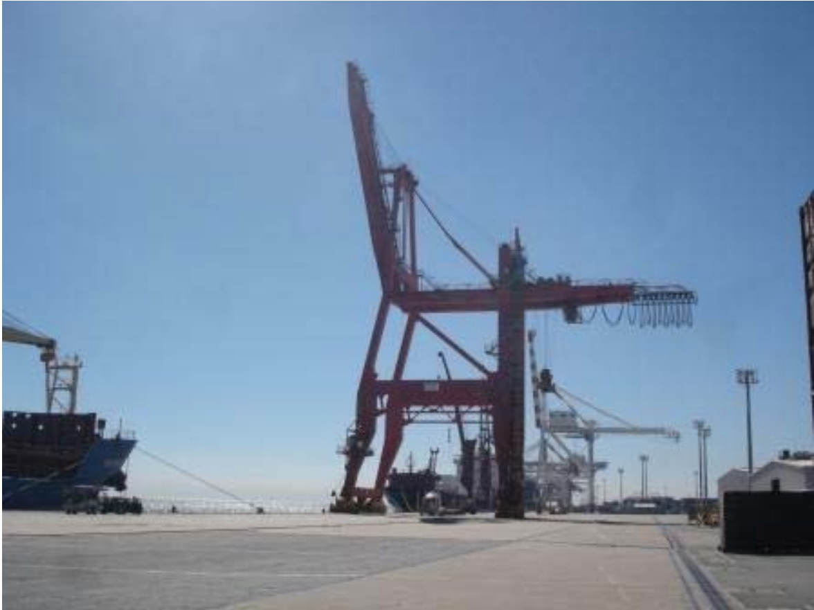
Picture 3 - Photograph of the Berth area at the FICT
