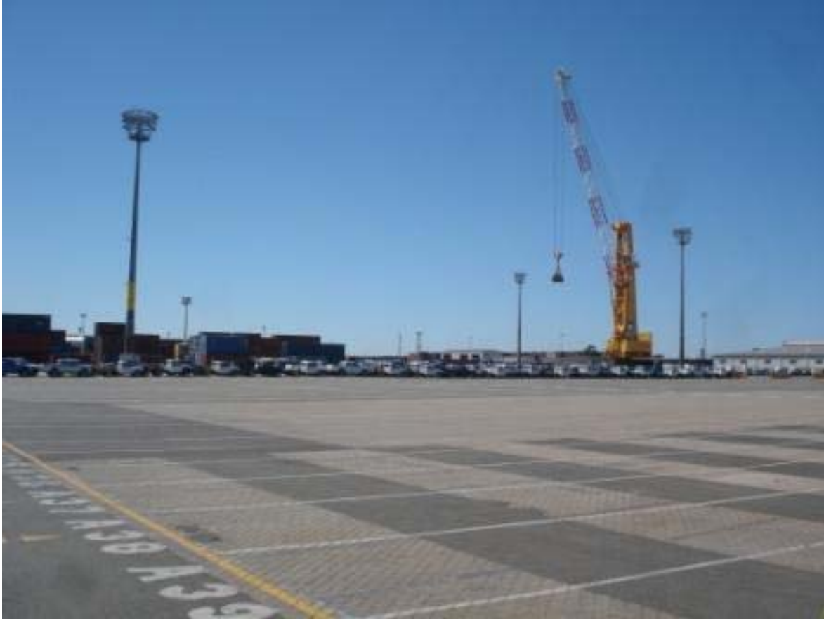
Picture 4 - Photograph of the temporary motor vehicle storage area and mobile crane
